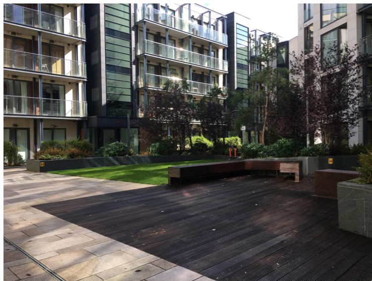
Figure 103: Grande Central apartments, September 2018
