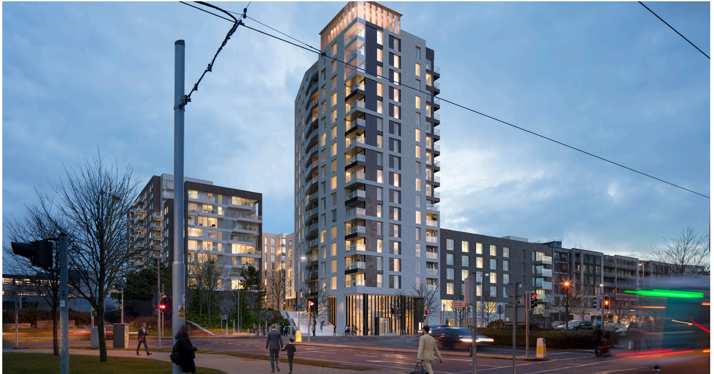
Figure 4: Photorealistic impression of the site as you can see it from the Luas stop
