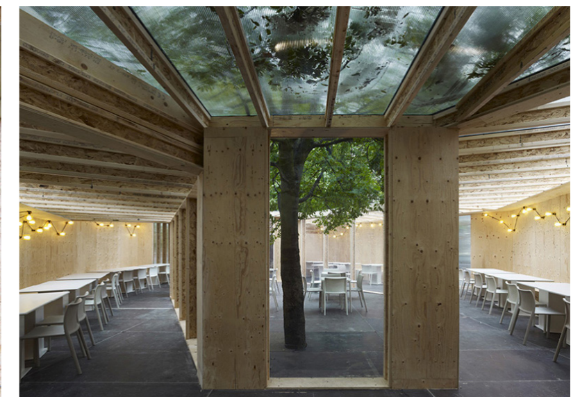
Figure 56: Timber pavilion with transparent roof for light penetration
